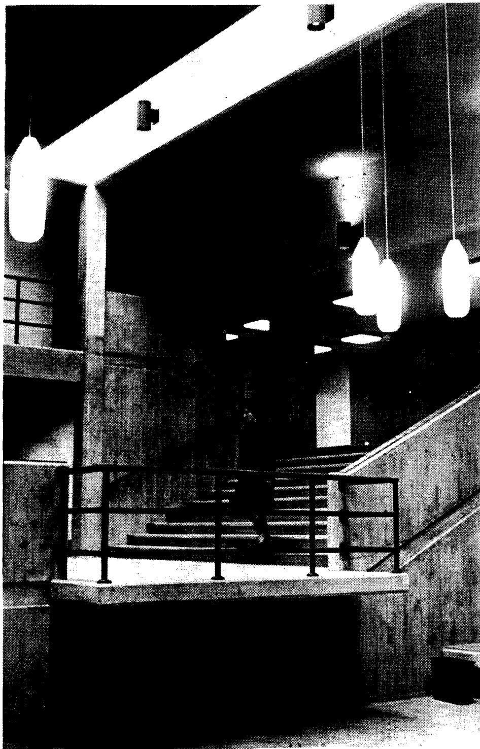
One of the solid cast concrete stairways leading down from the main floor to a lounge area outside the Fine Arts Studios.
